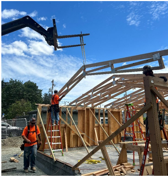
Truss being placed on addition.
