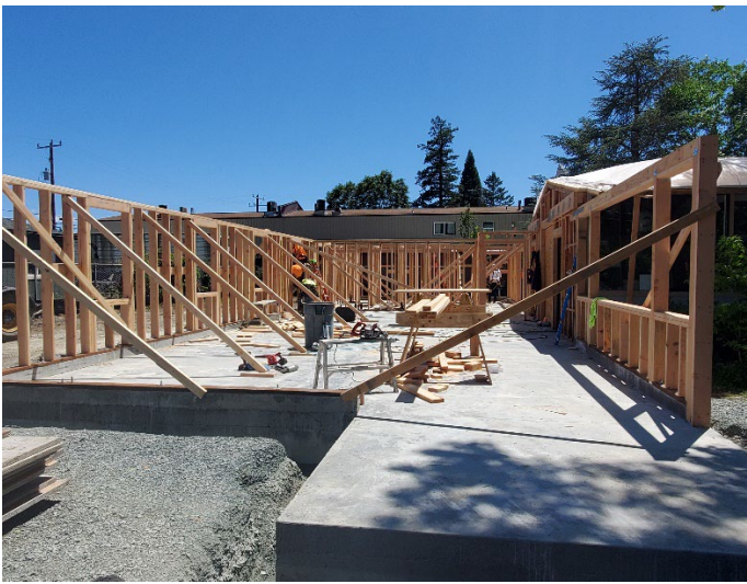
Exterior framing for library addition.
