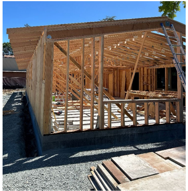
Trusses in place on addition.
