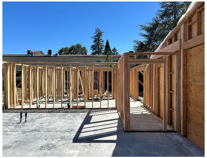
Framing for library addition.
