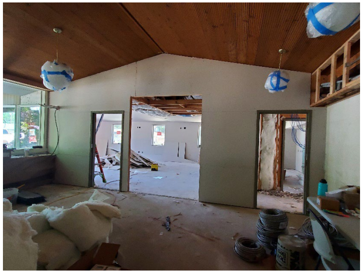
Doors from main library into addition, with drywall.
