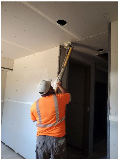
Taping the drywall.
