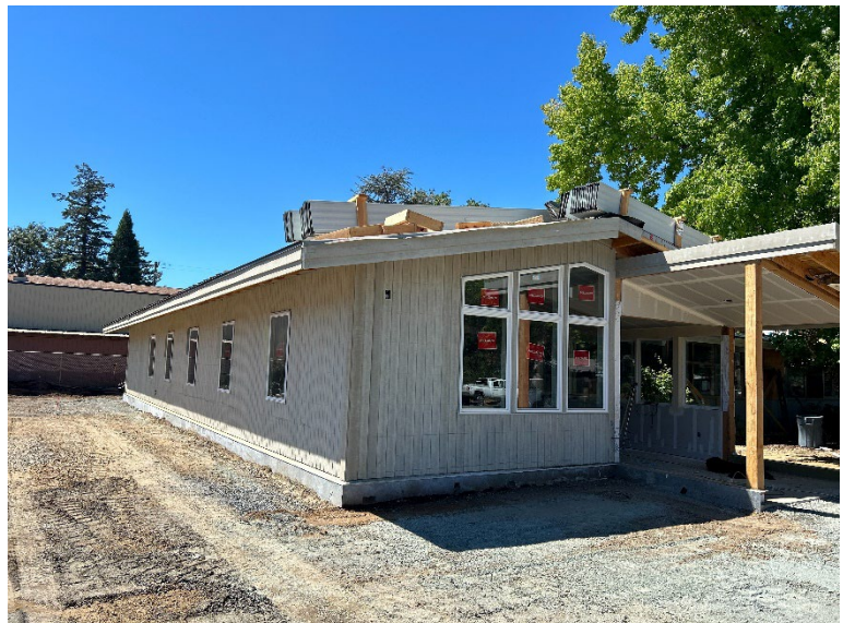
Addition with siding and windows.
