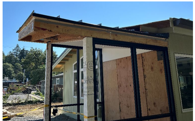
Community room vestibule.
