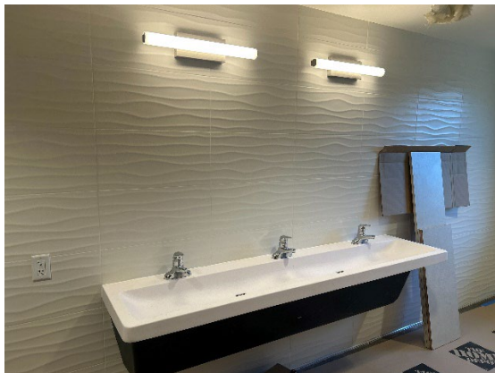
Addition bathroom sink and tiled wall.
