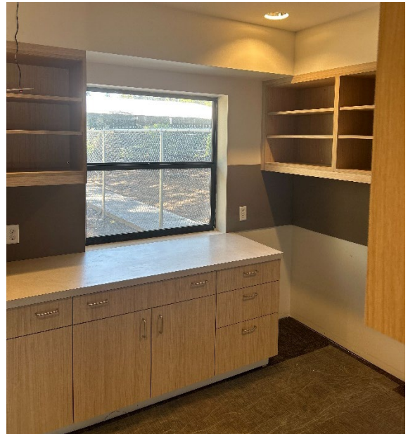
Back of house workroom with cabinetry installed.
